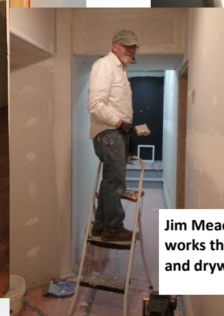
Left: You see the basement hallway leading from north to south outside of actors' dressing rooms and bathrooms. Insulation batting, drywall, mudding, texturing, painting and clean up is all being done by the lead team and volunteers stepping up to keep costs down as we finish the space under the exciting new reception hall expansion. Nearly 3000 hours of volunteer service have been given to the expansion. Many of the volunteers have excellent craftsmen skills; others of us are simply willing to offer helping hands. Often, that's just what's needed. The Laramie Plains Museum is very, very fortunate to have our network of volunteers—of all life skills and backgrounds—who step up when things need to be done. We could not do the wonderful things we do for this extraordinary historic property without our selfless, talented volunteers. Kudos to all!
